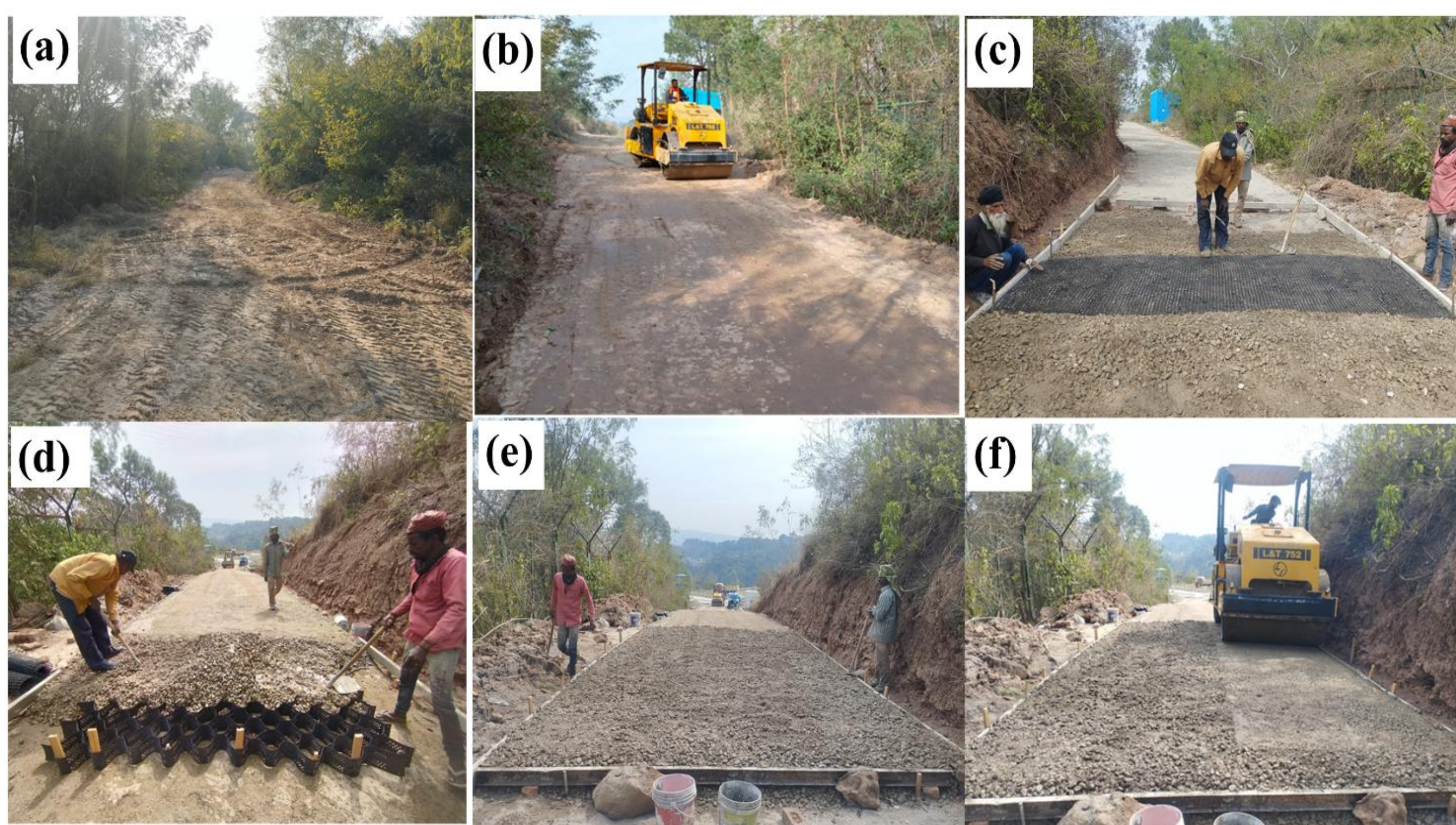
Construction sequence of test pit section: (a) Original subgrade condition, (b) Compaction of subgrade using roller, (c) Placement of geogrid in base layer, (d) Placement of geocell in base layer, (e) Base layer before compaction, (f) Compaction of base layer using heavy roller
